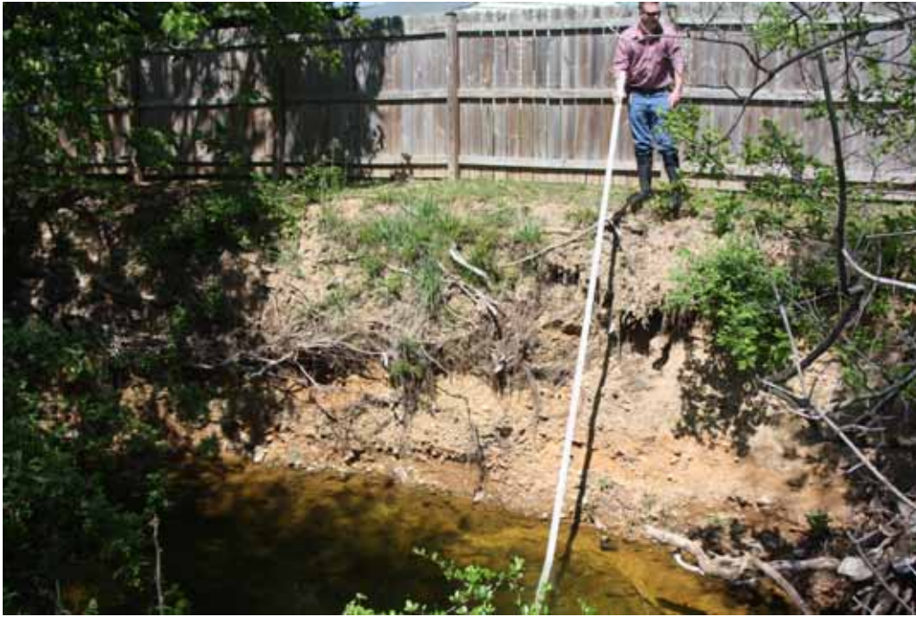
Figure 12 - Smithsburg Wastewater Treatment Plant site, (Urban Stream Restoration)
